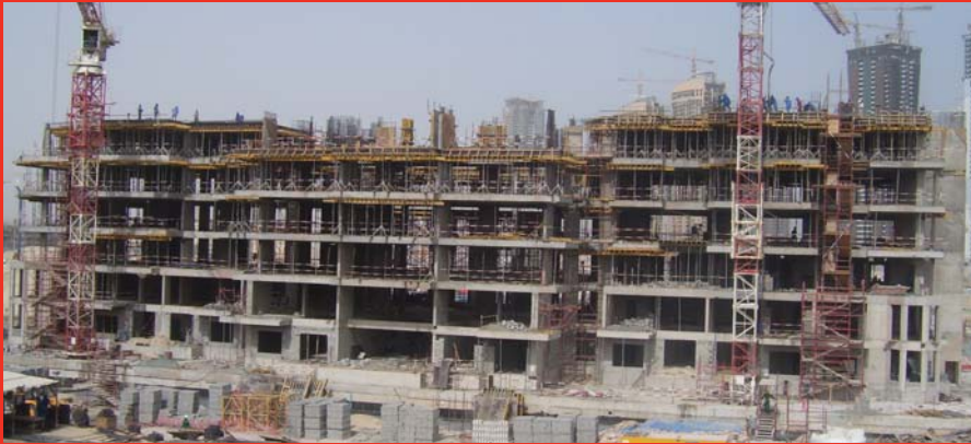
Clusters Building D – General View
