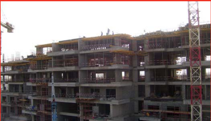
Clusters Building B – Roof floor slab on progress
