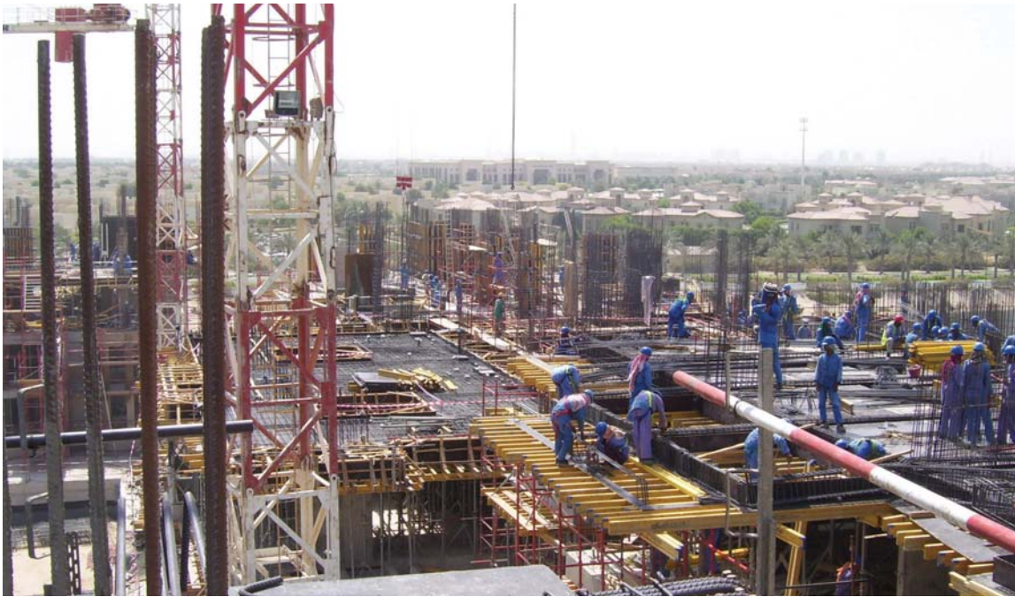
Clusters Building E – Rebars work
