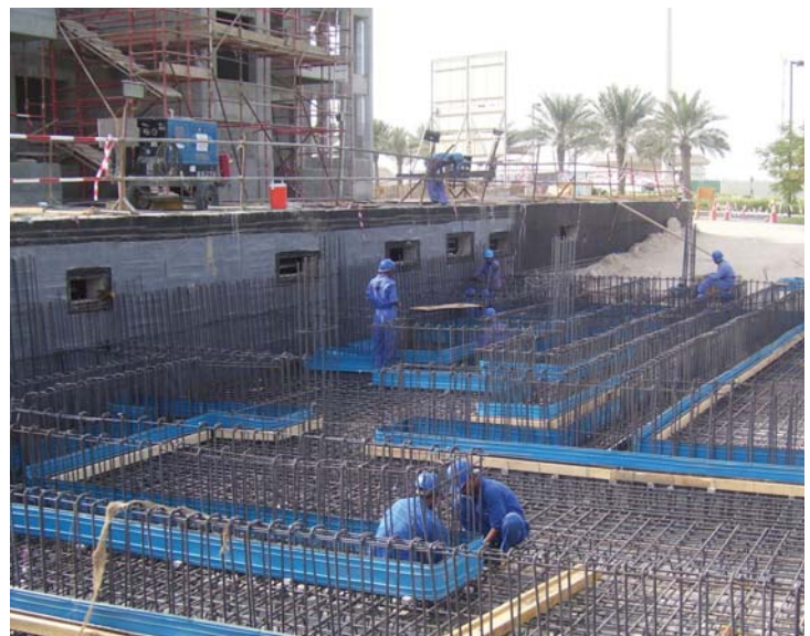
Substation takes shape
